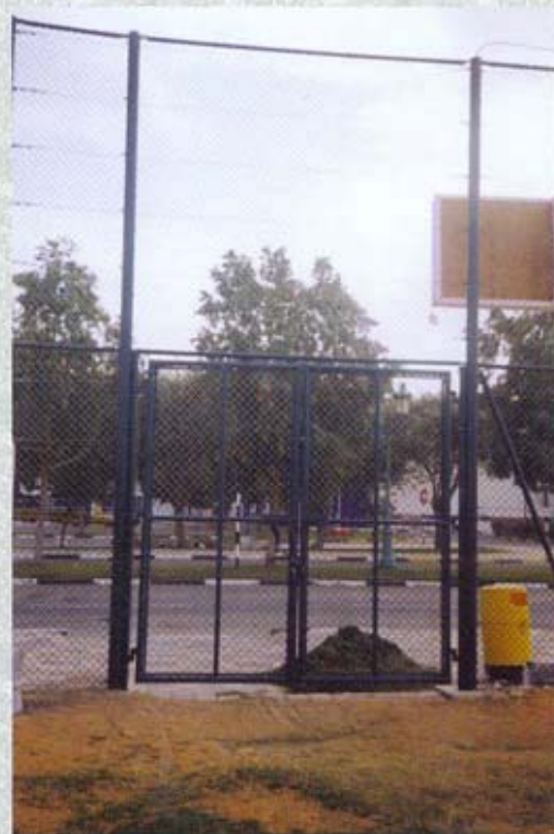
Gate for Tennis Court
